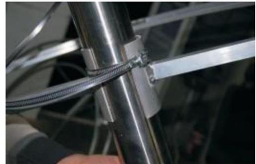
3. Where there is an opening in the guide, drill through the long arm of the fastening support, to screw the arm and the guide together.
